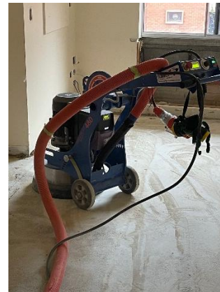
Three floor grinders are currently in operation
