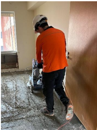
The floor grinder removing glue from old floors
