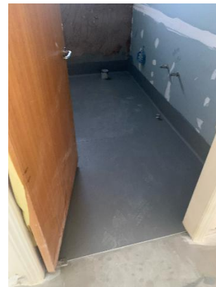
Floor screeding in the bathrooms
