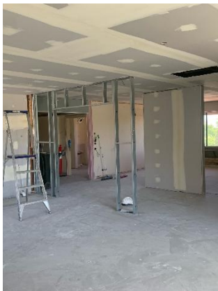
Completed repairs to walls and ceilings
