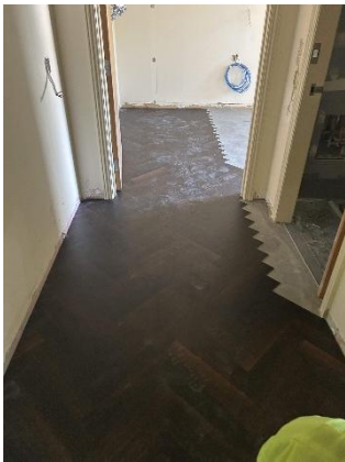
New flooring in progress
