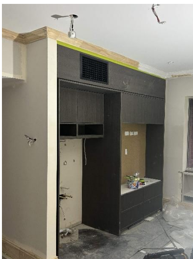
Kitchen cabinetry being installed
